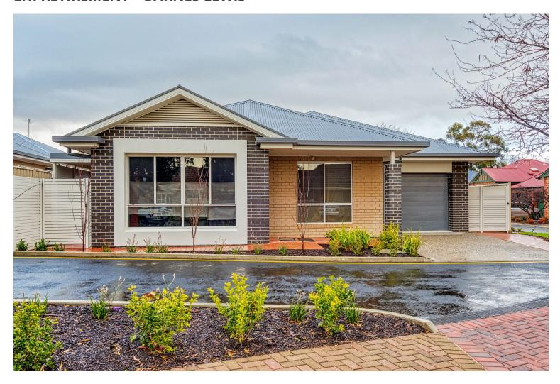
LHI Retirement Barnes/Lewis was the construction of six new 3-bedroom residential dwellings, a new 300m2 maintenance facility as well as the associate driveway and landscaping works. The steel framed brick veneer dwellings were designed for independent living including DDA fixtures and reinforced walls. The project was surrounded with feature brick fencing and security auto-gates to create a gated community.
